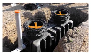
The Endura XL Safety Strap is an optional attachment to any Endura XL Interceptor: past, present and future! The device may be assembled during new installations or added to any Endura XL Interceptor currently in operation. Detailed installation instructions are provided with the kit. The Endura XL Safety Strap provides an added level of protection to workers during cleanouts and to the public at large.
